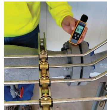
At the most recent install, the city gate station is recording 82-85 dBA at approximately 1600 MCFH with a goal to stay within 90 dBA at maximum flow rates of 2200-2500 MCFH during colder months.
