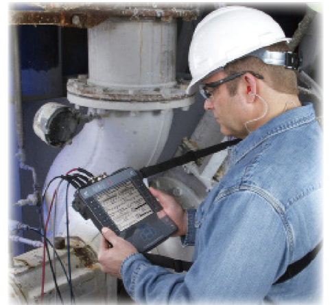
Vibration data collection using AMS 2140
