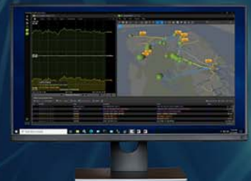
Monarch SCADA Platform
